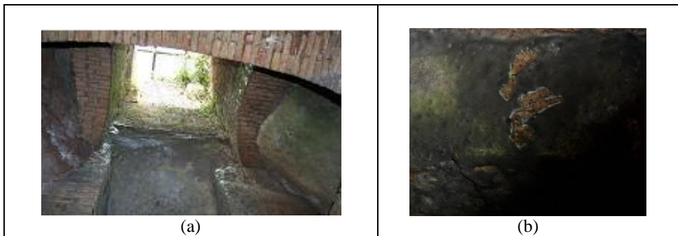
Figure 8. (a) The general aspect of skylight where phototrophic biofilm and vascular plants were developed, (b) and a detail of the sample area of the phototrophic mat, where a white layer was observed beneath.
