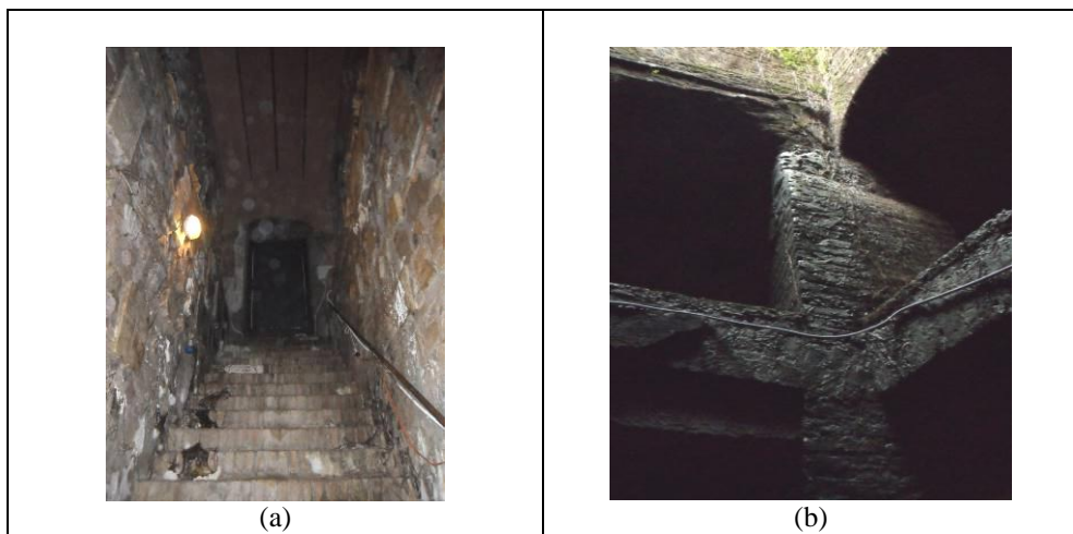
Figure 3. (a) The biological colonization at the entrance chamber (entrance door in the background) of the catacomb and (b) on the walls located near the skylight.
