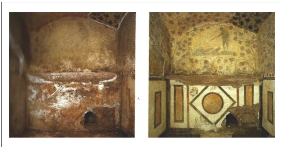
Figure 4. Vatican Necropolis, Mausoleum M, interior north wall with the Christian figure of the fisherman before and after restoration (from [3, p. 113], ©Fabbrica di San Pietro). Soluble salts are clearly visible before restoration.
