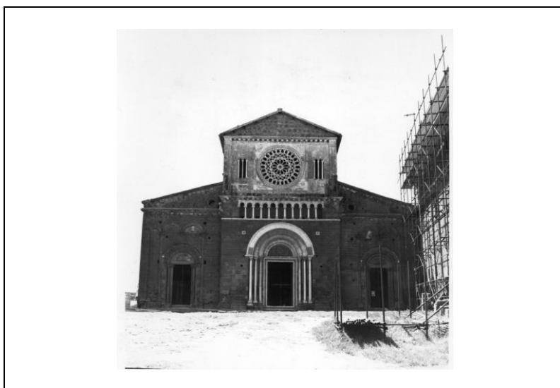
Figure 7. Restoring works of Saint Peter Church in Tuscania after the 1972 earthquake by Antonio Gentili (called Toto, 4 th generation).
