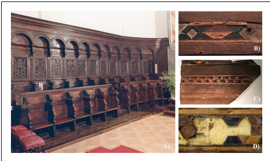
Figure 1. The wooden choir of San Rufino in Assisi: (A) Choir with bas-relief panels and pillars (photo Saccumani), (B-D) motifs realized by means of the inlaid ‘a toppo’ to hidden joint by nails. Note the nail and the paper layer in (D).
