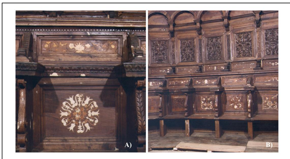
Figure 3. (A) Grouting in the decorated parts of the inlays and in the frames, (B) the choir during restoration (photo R. Saccuman).
