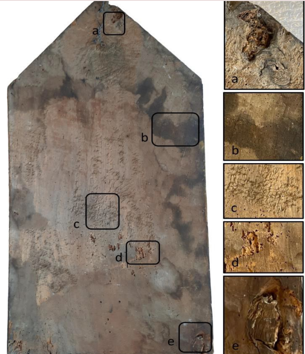
Figure 2. Rear of the wooden support. Details of the observed defects: (a) and (e) - knots, (b) discoloration, (c) truncated fibres, (d) damage caused by entomatic galleries.
